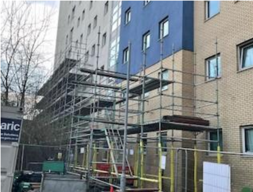
Phase 4 scaffolding ongoing
